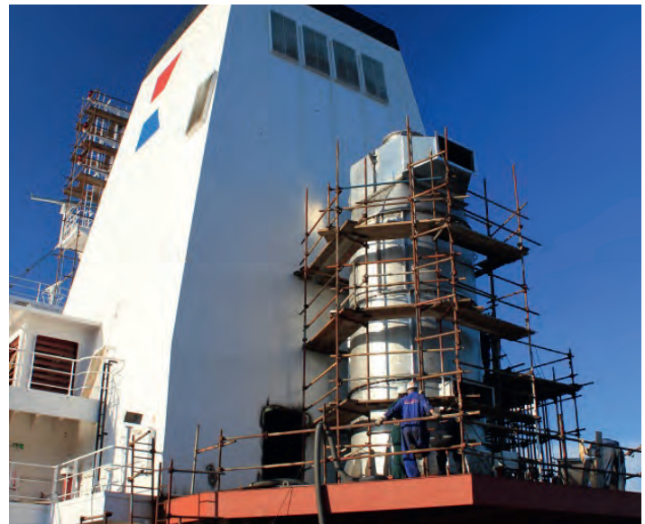
Conversion: The SAACKE wash tower was installed directly behind the stack.
